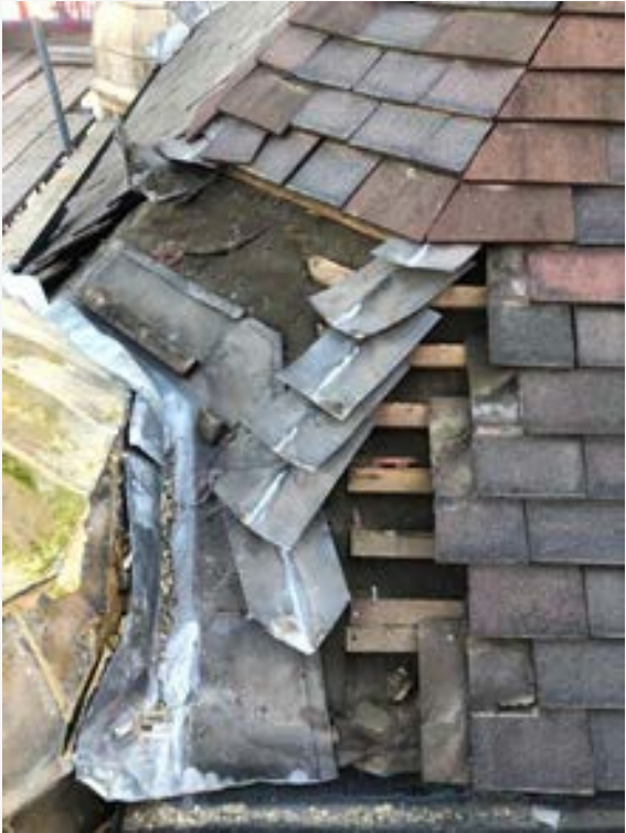
Damaged roof coverings and guttering | Loose and missing roof tiles
