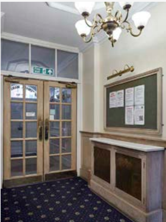
Dirt stained and bulky radiator casings | Untidy appearance from clutter and poor signage | Inefficient bulbs (previous frequently blown)
