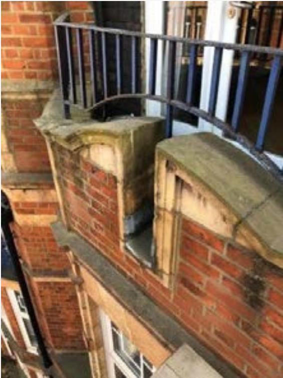
Stained and damaged details to facade | Multiple layers of peeling paintwork to railings
