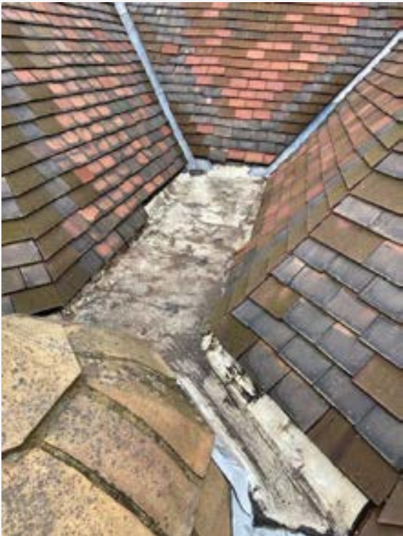
Damaged roof coverings and guttering
