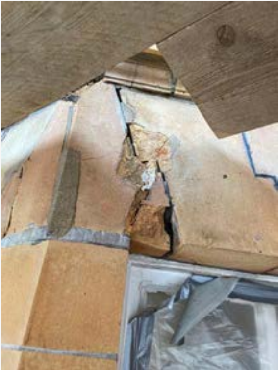
Cracked and damaged masonry
