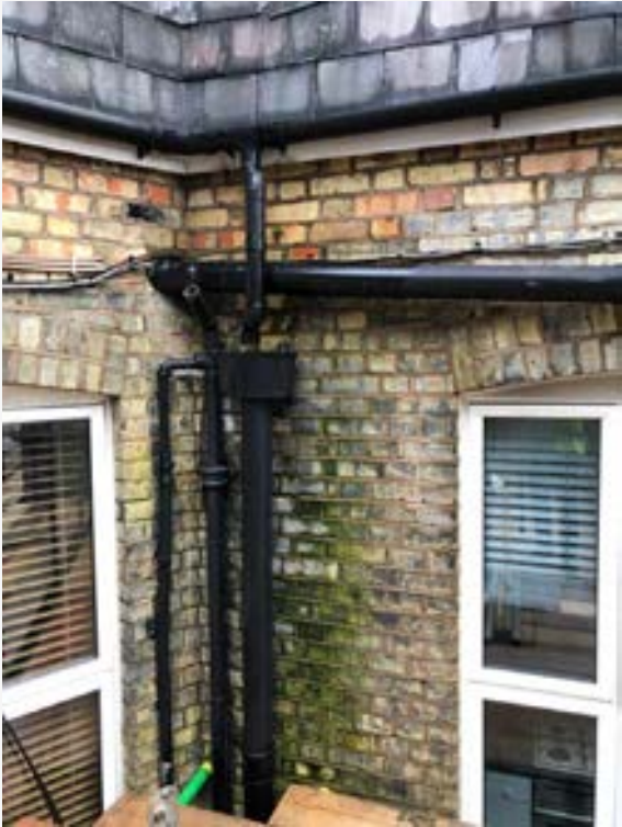
Leaks leading to brickwork staining
