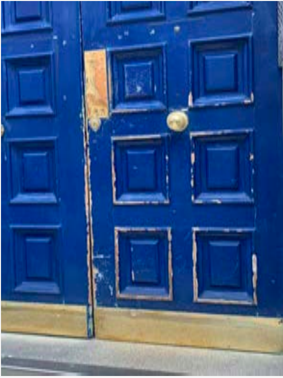
Continuously chipped paint finish to doors
