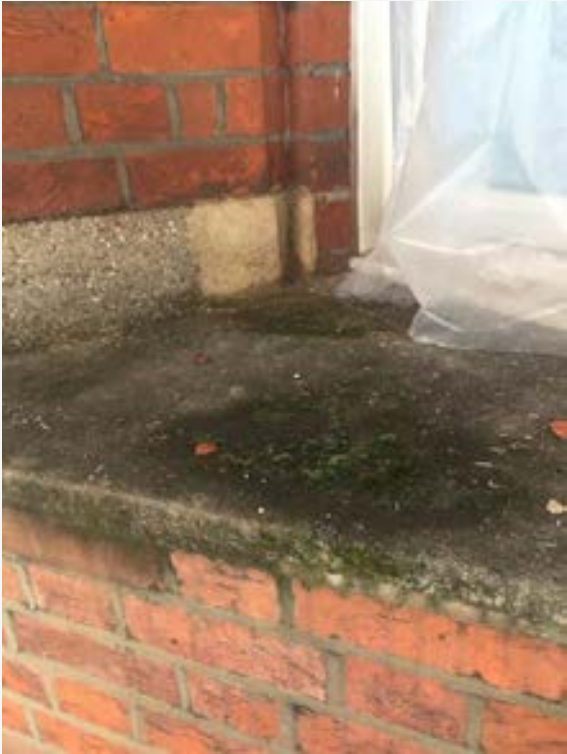
Water damage to window sills
