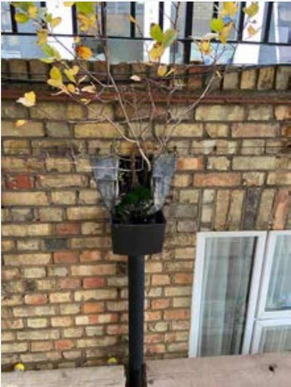
Blocked and undersized rainwater goods
