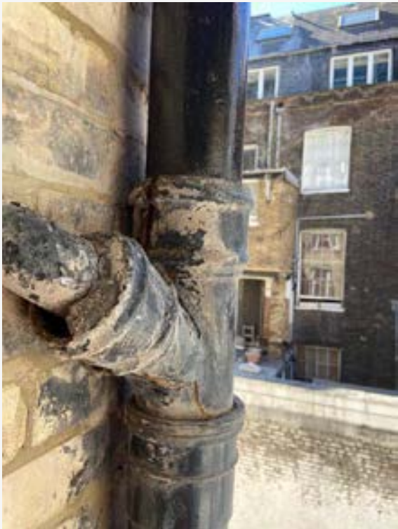
Corroded rainwater goods
