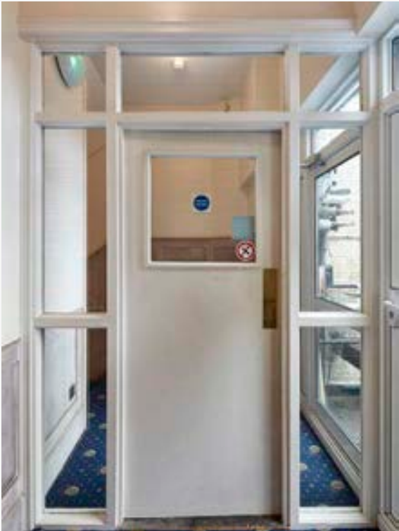
Fire doors with excessive gaps and of poor appearance and inconsistent finish throughout
