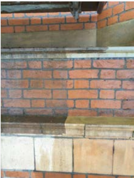
Progress during cleaning of brickwork
