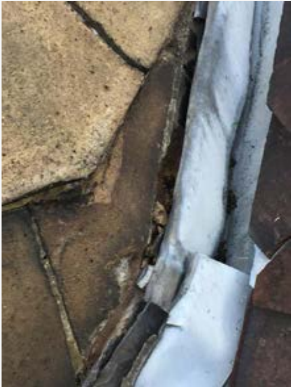
Damaged roof flashings
