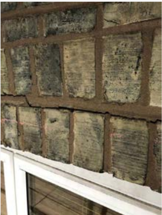
Poor brickwork repairs and previous re-pointing
