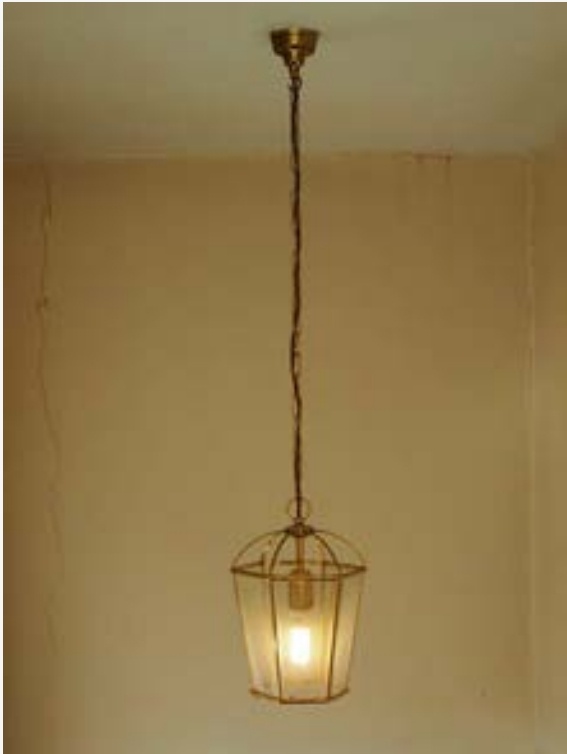
Poor lighting levels | No lighting control and energy inefficient fittings
