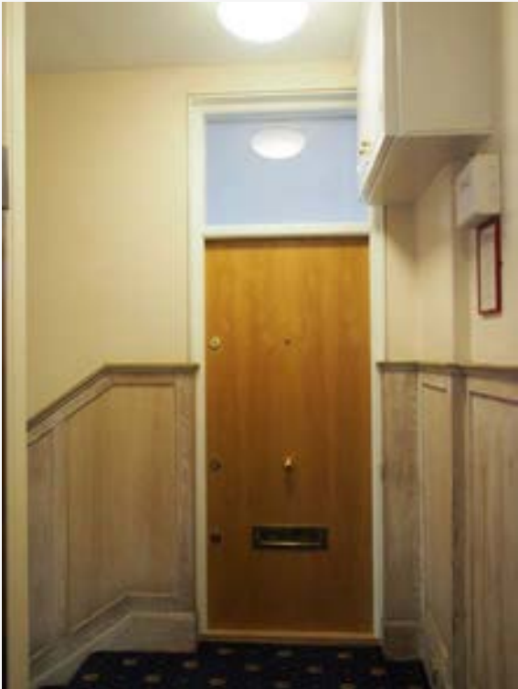
Fire rating of doors unverified and without self closers | Inconsistent appearance
