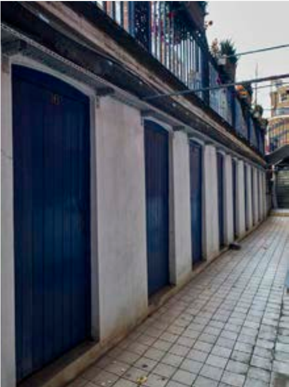
Redundant wiring | Broken floor tiles | Stained paintwork | Vault doors water damaged
