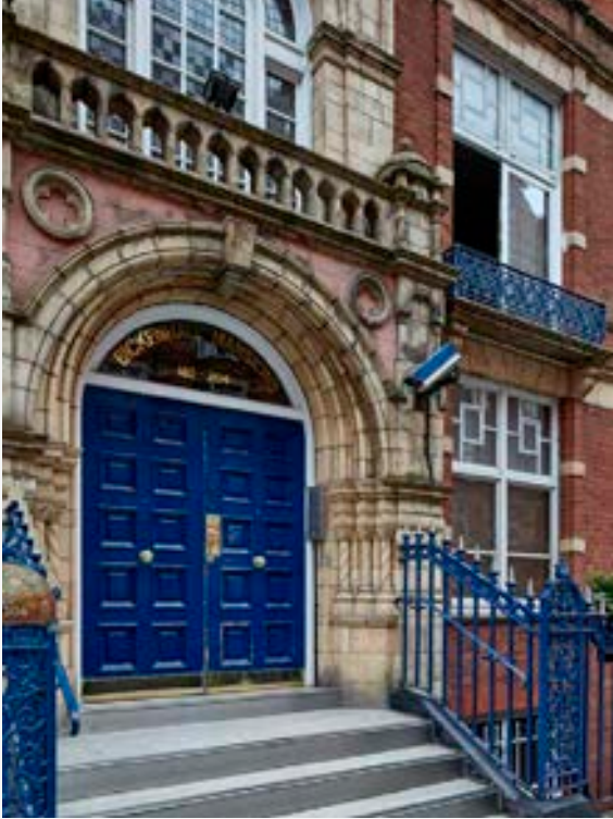
Low quality floor finishes | Exposed cabling and wiring | Oversized CCTV | Stained masonry and terracotta
