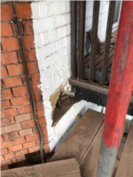
Corroded steelwork and missing pointing in foreground to brickwork
